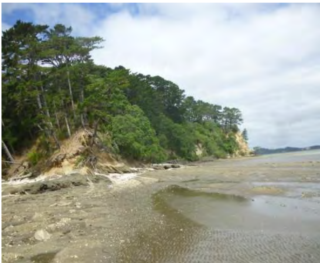
Figure 104 Coastal erosion, 2014, Source: Auckland Council Heritage Unit
