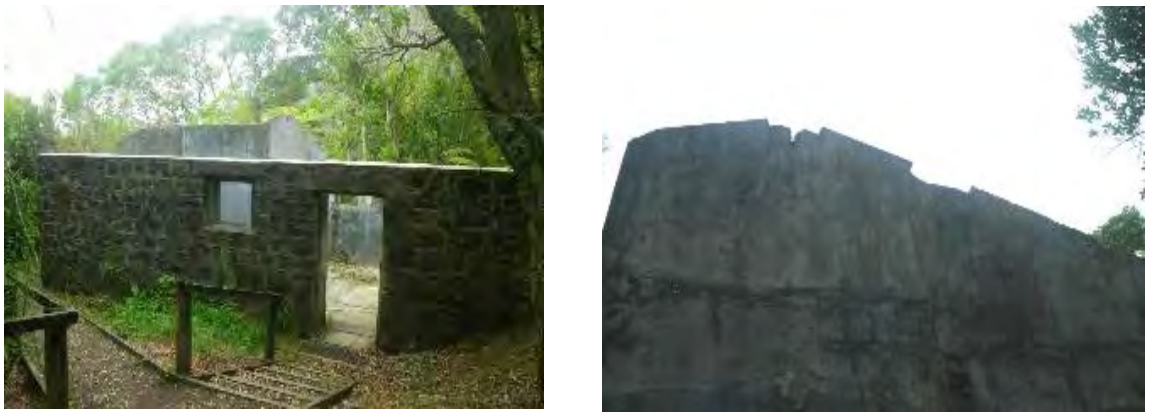
Figure 111 Entrance to building and wall supporting the roof, Source: Auckland Council Heritage Unit
