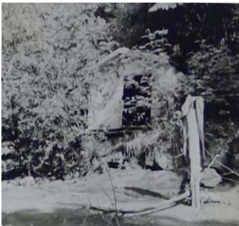
Figure 116 Shed 3 (1971) D.A. Davey, 23 Albrecht Ave, Mt Roskill. Source: Auckland City Archives
